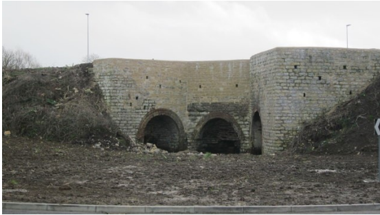
Limekiln Roundabout on the Junction of the A38 with the newly opened South Bristol Link
